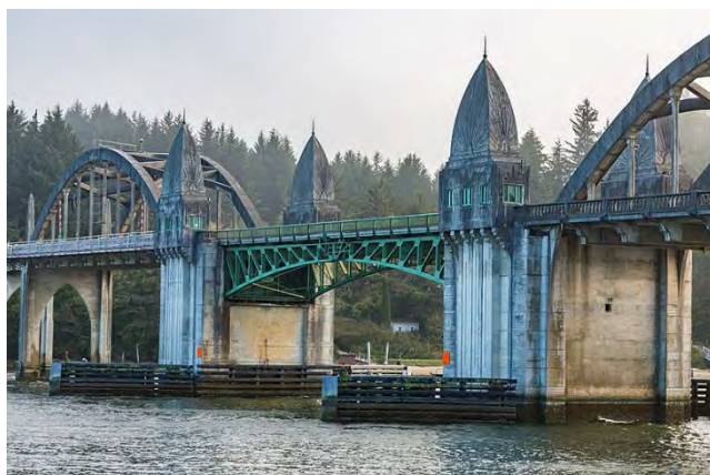
Historic Siuslaw River Bridge over the Siuslaw River, as seen from Florence, Oregon | Photo by Tony Webster via Wikipedia Commons
