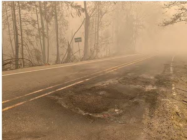
Damage along OR-126, McKenzie Highway during the Holiday Farm Fire (2020) | Source: Oregon Department of Transportation
