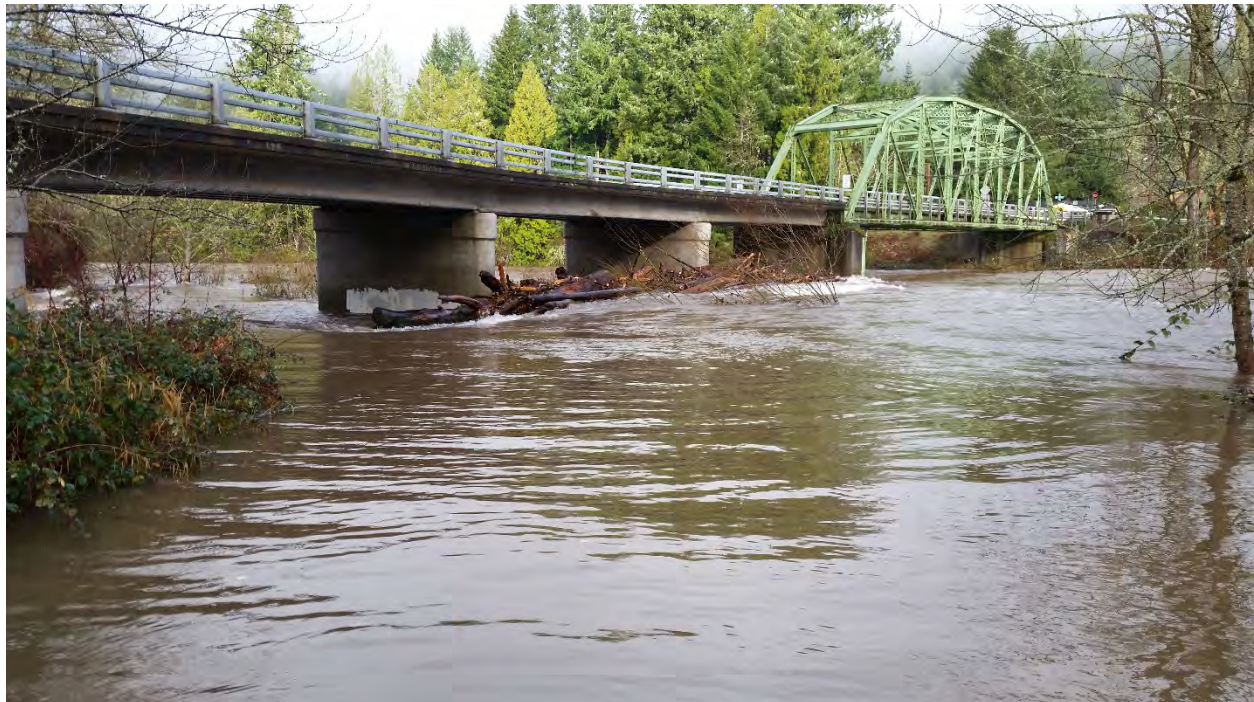
Bridge Street bridge experiencing rising waters and debris during a December 2014 event. | Photo: Lane County Public Works, Roads Division
