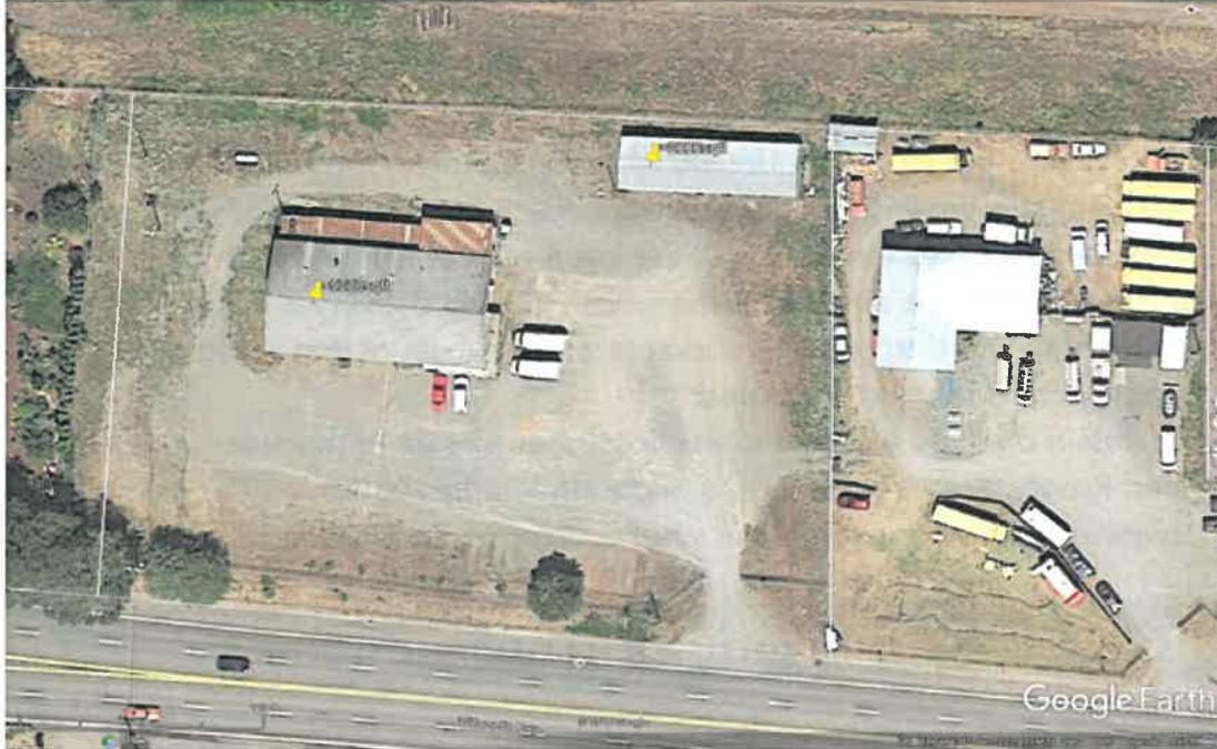
Figure 7: Public Works Building for Phase I Use
