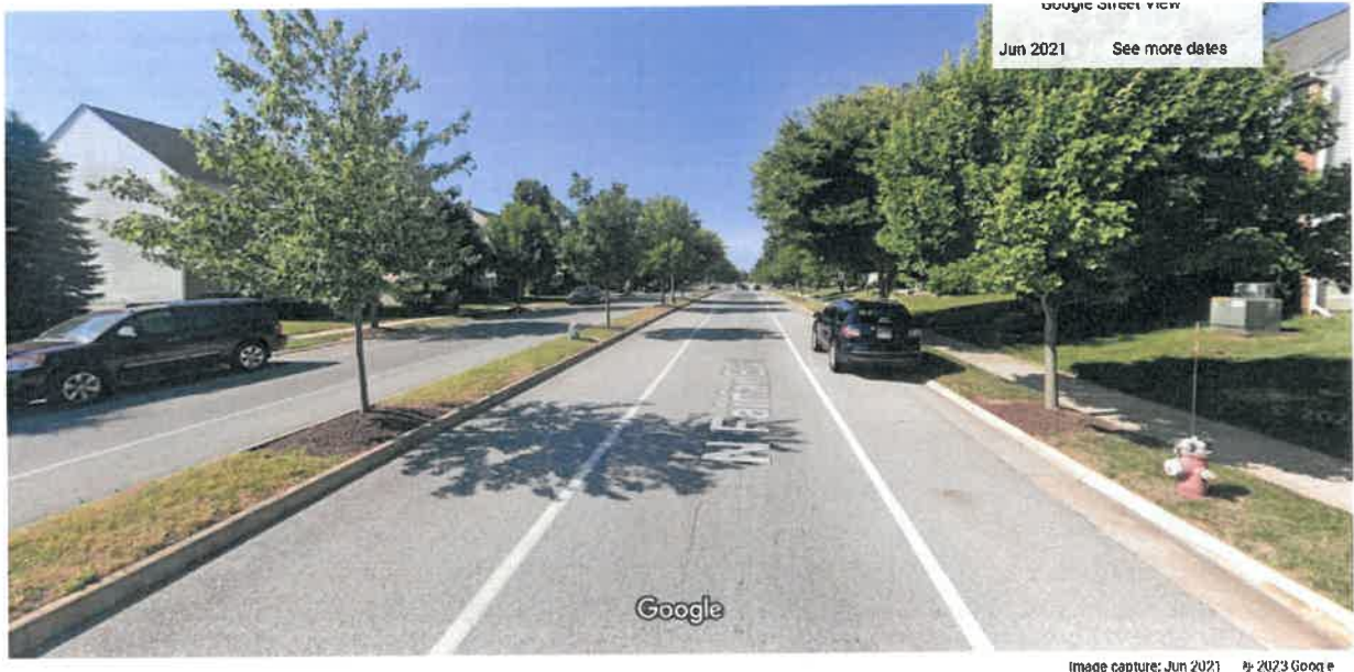
North Fairfax Boulevard after the parking lanes were painted and street visually narrowed. (Source: Google Maps.)
