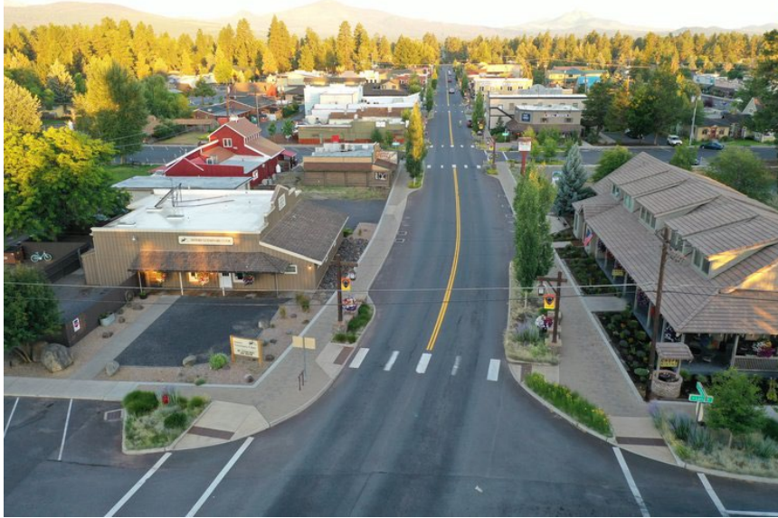
Figure 5. Streetscape Improvements in Sisters, OR including street trees, curb extensions, and bioswales.
