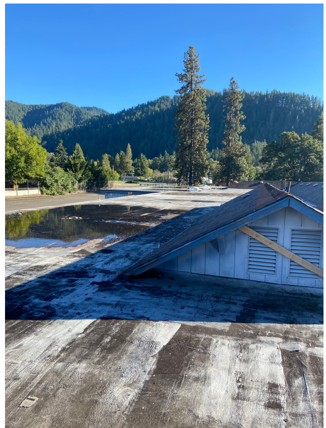
Figure E. “Penthouse” roof structure
