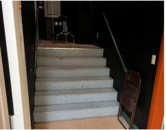
The stage is located at an elevated level as well. The building code will not mandate providing access to the stage as a base requirement for improvements of Module C, but use of the stage should be evaluated for ADA compliance and risk to the city. Options to access the stage, including motorized lifts should be evaluated. For reference, the stage is slightly more than 44 in. above the gym level, therefore a ramp of more than 44 ft would be required.
