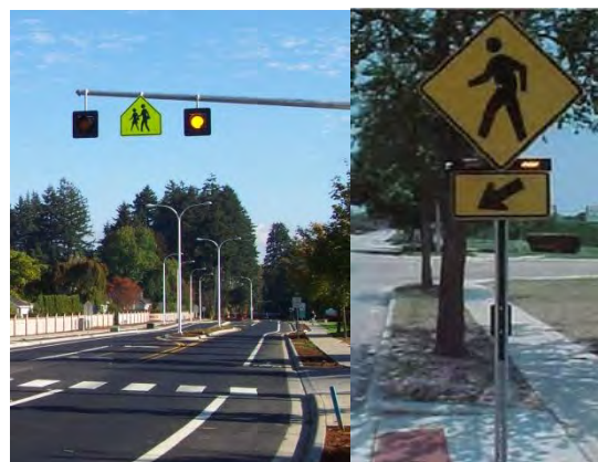
PEDESTRIAN TOOLBOX EXAMPLE TREATMENTS (ON LEFT: OVERHEAD FLASHING BEACON; ON RIGHT: RRFB SIGN ASSEMBLY)
