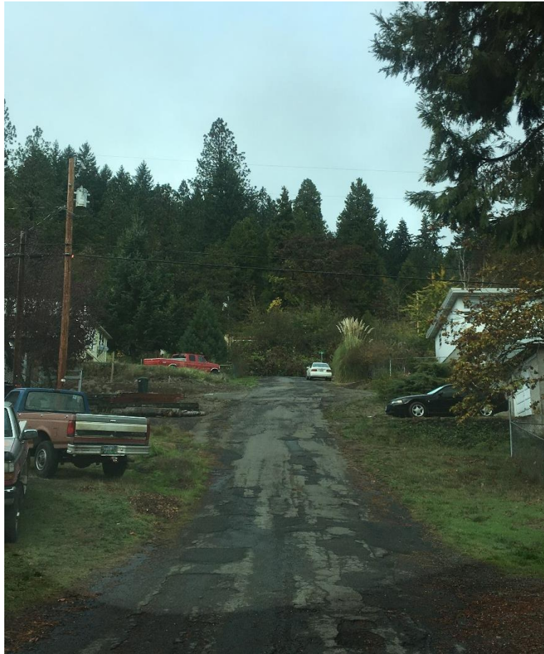
Example of roadway in need of repaving
