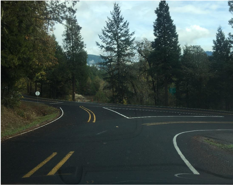
Figure 13B Streetview of Westoak Road/High Prairie Road facing east from Westoak Road
