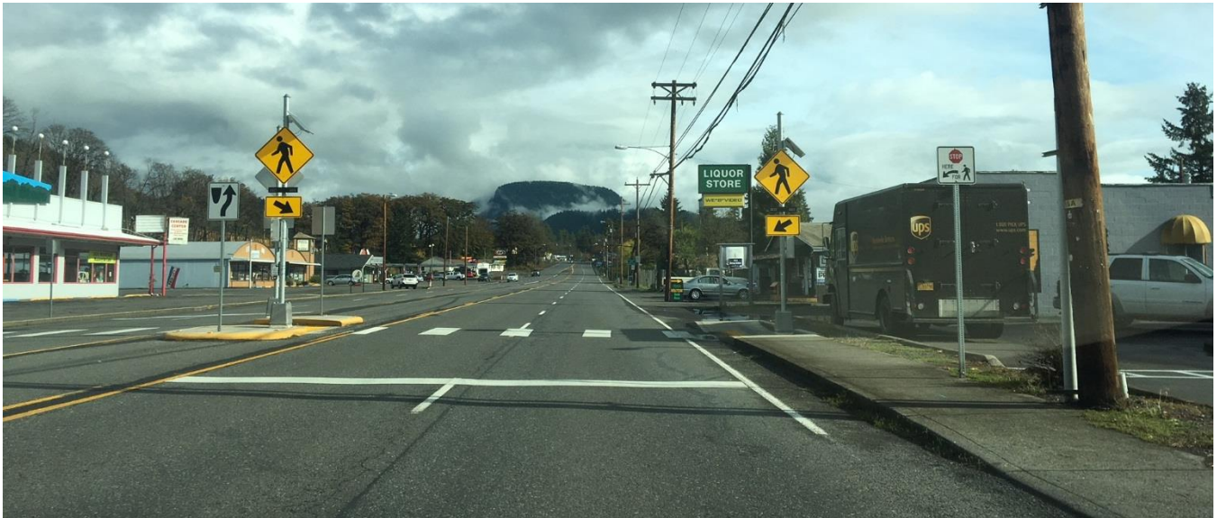
Illustration of Pedestrian Crossing with RRFBs Installed on OR 58, West of Rock Road
