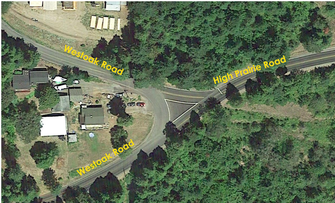
Figure 13A. Aerial of the Westoak Road/High Prairie Road Intersection
