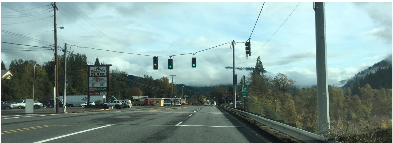
Illustration of existing crosswalk at OR 58/Crestview Street that lacks a sidewalk or shoulder for pedestrians on the south side of OR 58.
