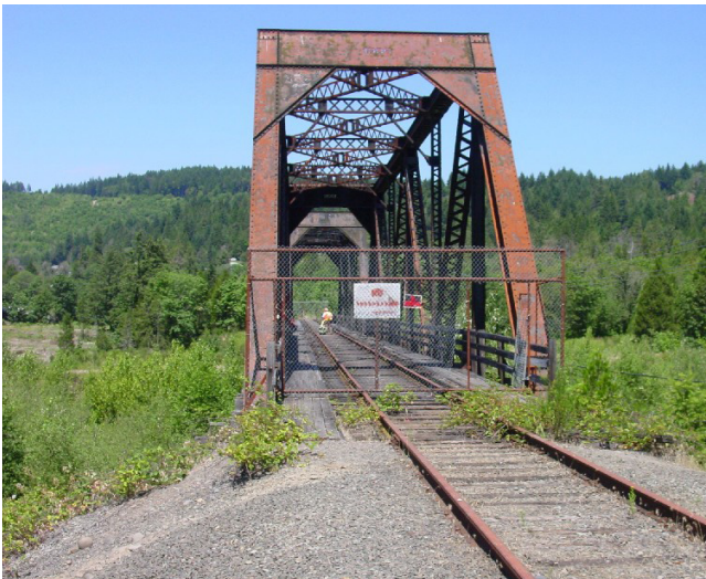
Old railroad bridge
